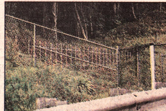
Rows of bars keep debris from overloading the chain link fence along the H-3.
